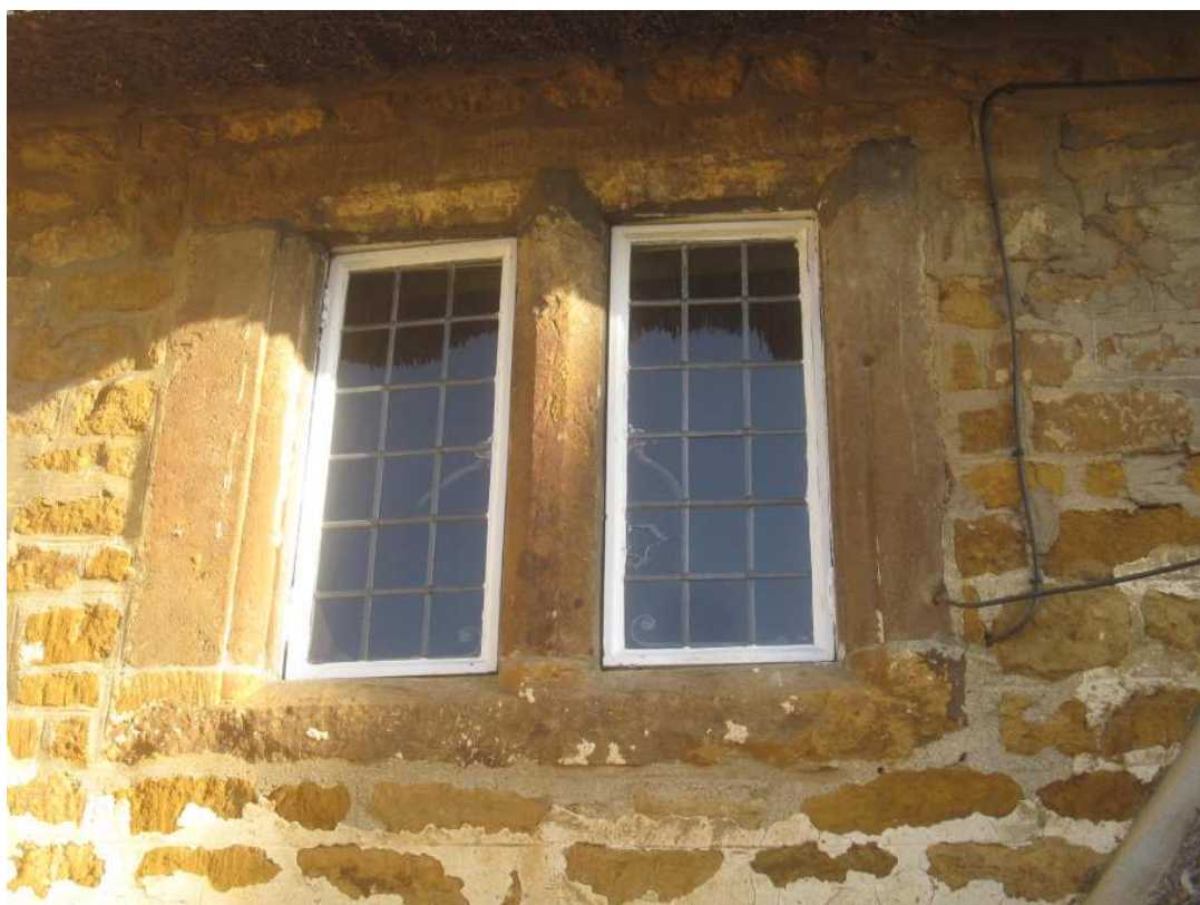
Rear first floor window, with ovolo-moulded jambs and chamfered mullion
